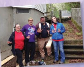
The Walgreens Team constructs new raised garden beds at Daily Bread
